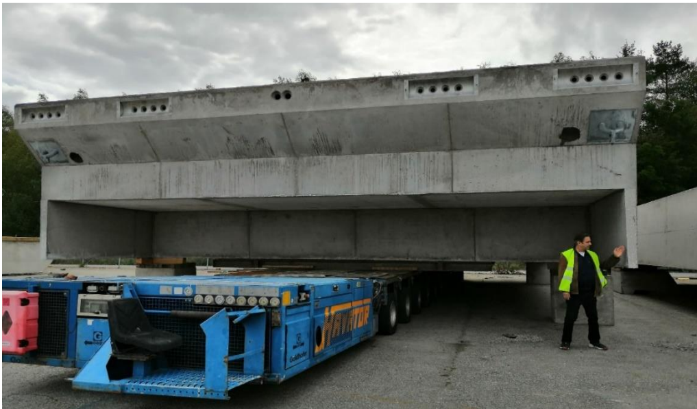
Figure 7 The 190 tons heavy wave breaker from Pontona (august 2019).
