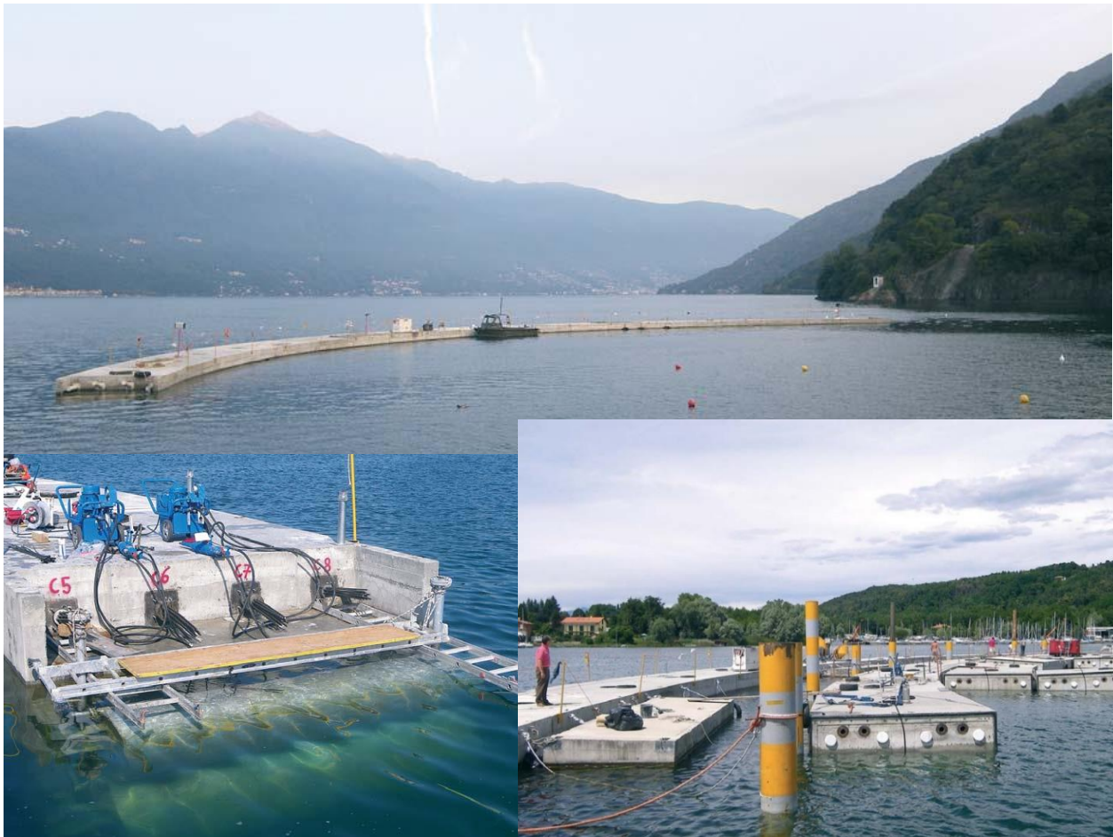
Figure 2 Example of pre-tensioned float quay from Switzerland.
