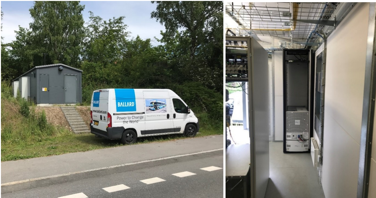
Figure 29 - Hybrid system installation
