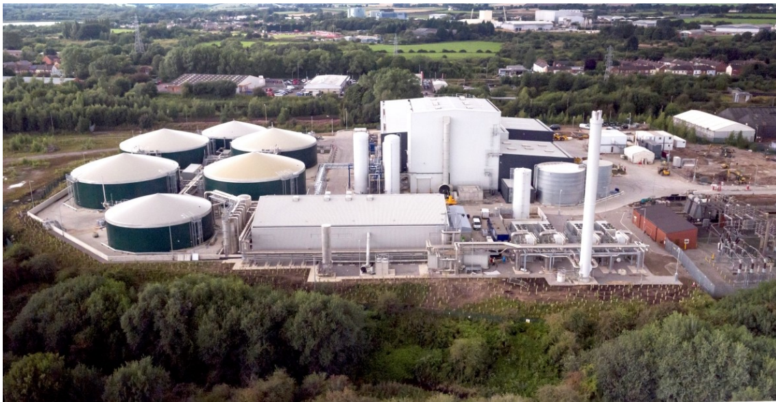
Figure 3 the plant subsequent to second milestone, full installation process was done and ready for handover.
