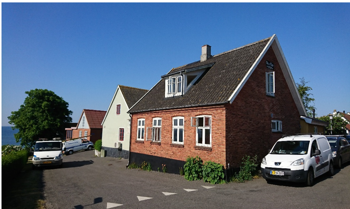
Arnager house before BIPVT modules
