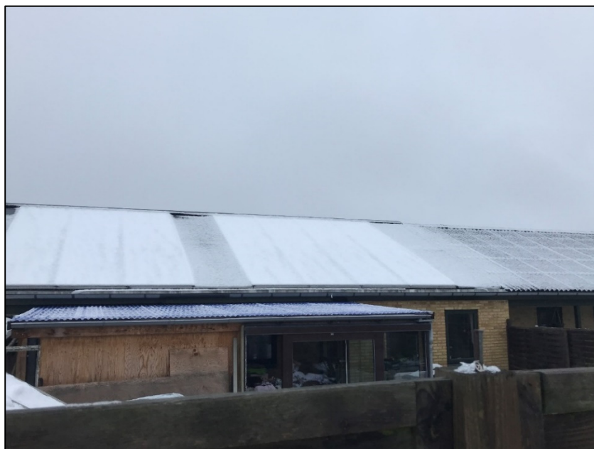
The areas without snow are with modules that do not have built-in insulation layer
