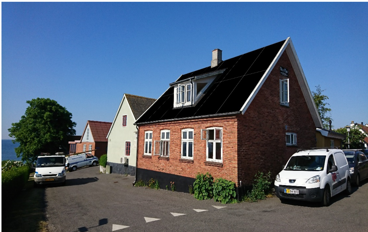
Arnager house after BIPVT roof modules
