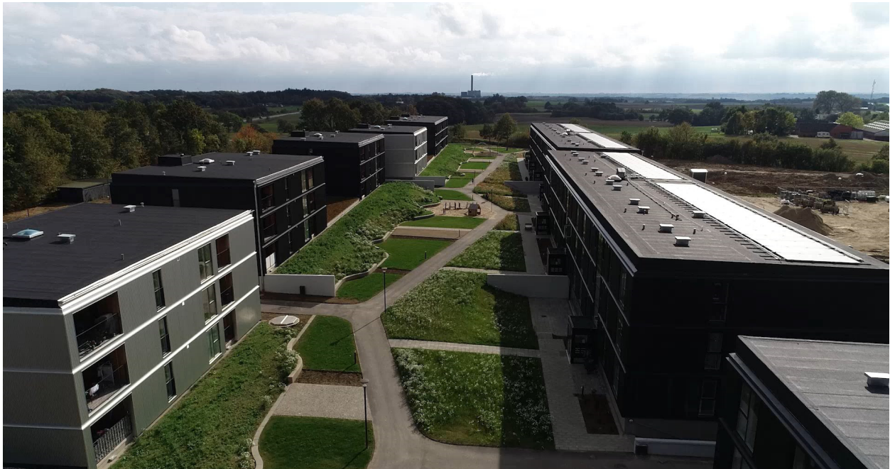
Figure 3.2.1 (III) the PVT-E system on three building blocks in Århus
