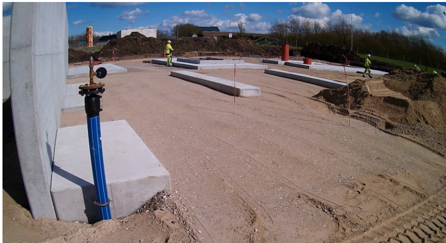
Figure 1: Hybalance site - foundations completed
