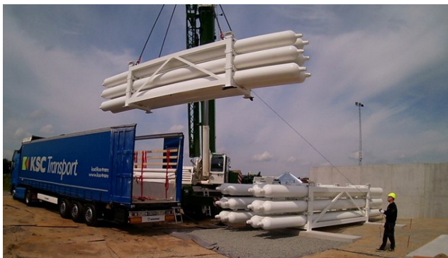
Figure 2 : Delivery of the equipment on site
