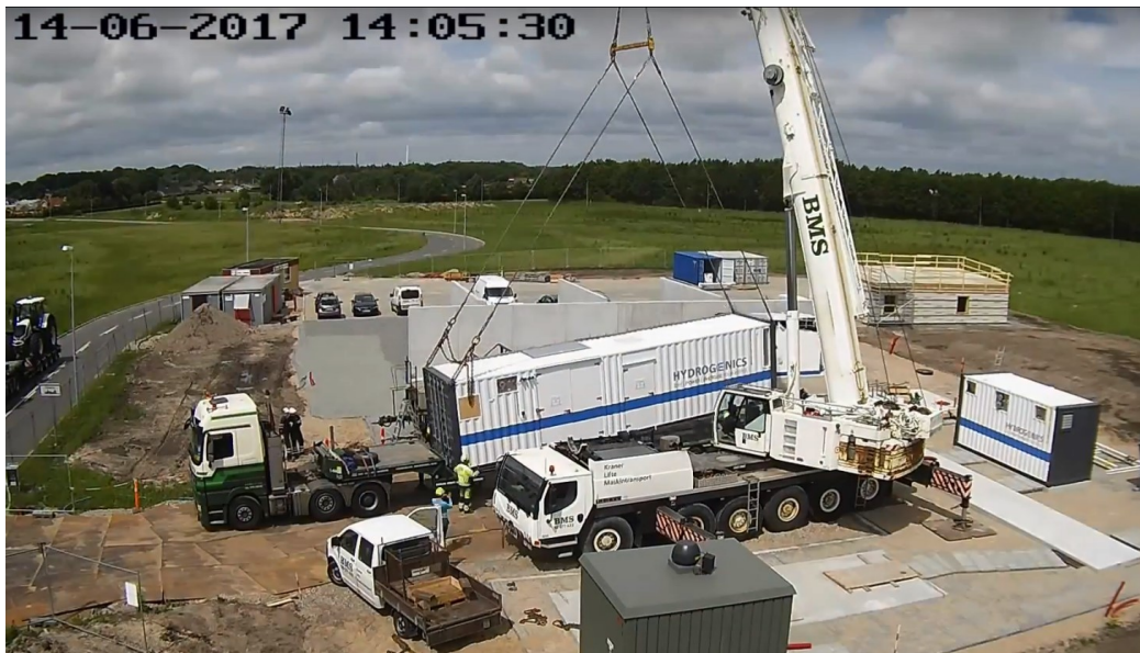
Figure 7: Installation of the electrolyser in the Hybalance, Hobro, Denmark
