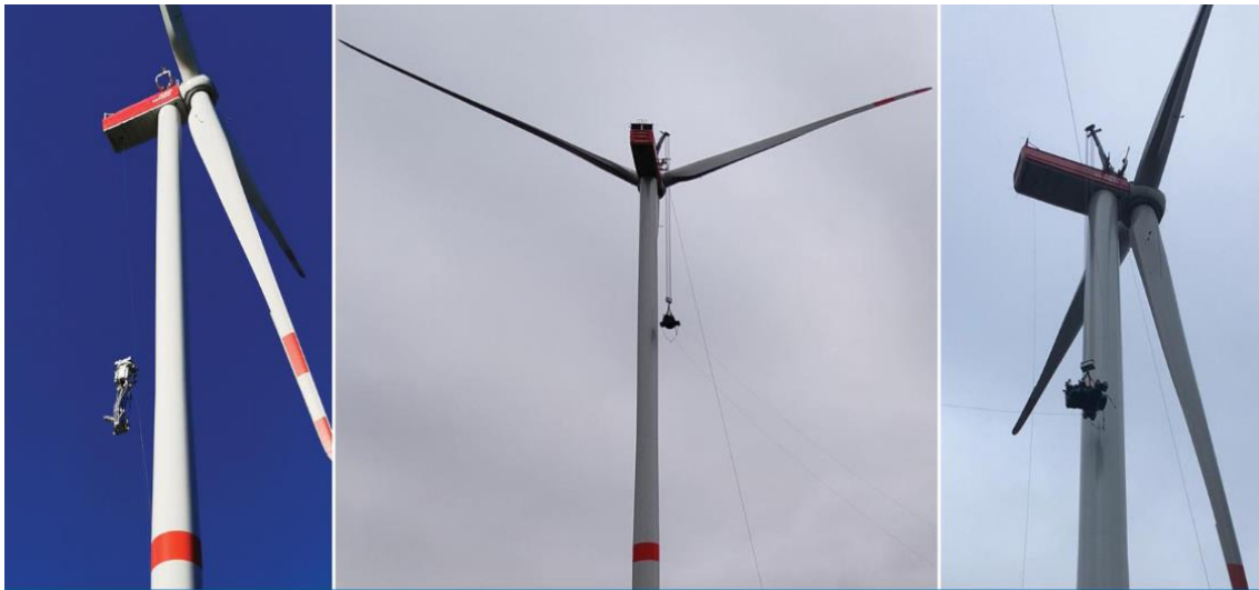
First test of the on-shore version of the crane
