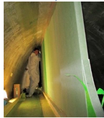
Figure 12: A) and B) Prototype #1 and #2 are both designed to be retrofitted in a SSP34m blade. For each prototype, experience is gathered and used in the design for the next prototype. C) The Floor™ prototype are retrofitted in the LM58.7m blade which are almost twice as long as the SSP34m blade.
