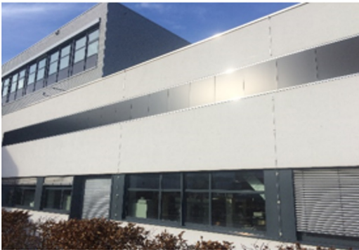
Mittag et al (2016) TPedge: glass-glass photovoltaic module for BIPV-applications
