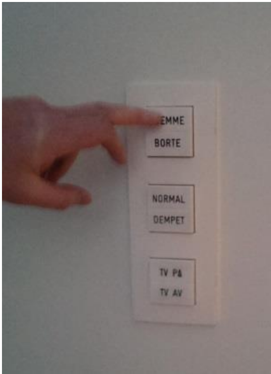
Figure 23. Smart grid solutions can be very simple, but still popular (the labels state: Home/Away, Normal/Reduced, TV set on/TV set off).
