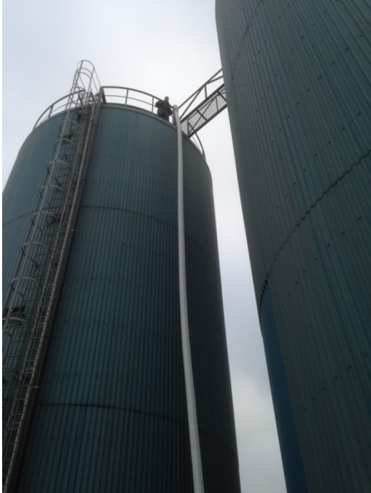
Figure 17 Sampling of leaking gas at the top of a biogas reactor
