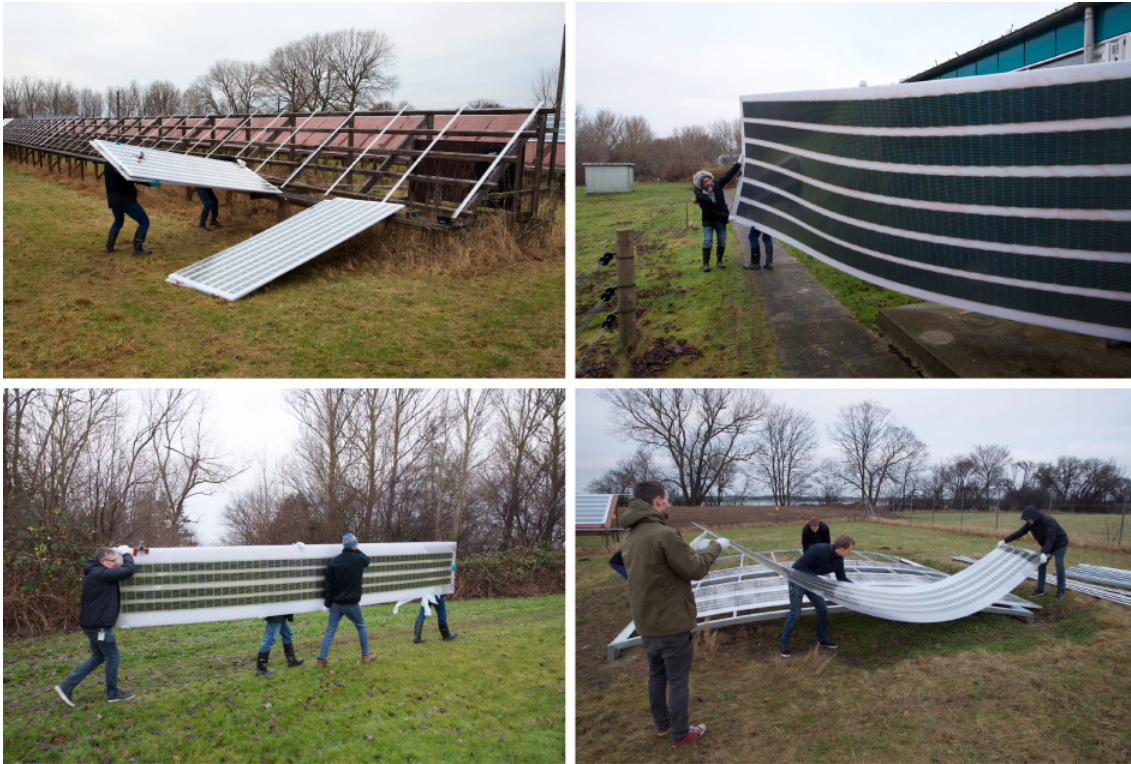
Fig 9 Solar roof plate panels are lightweight, flexible and fabricated in various sizes.
