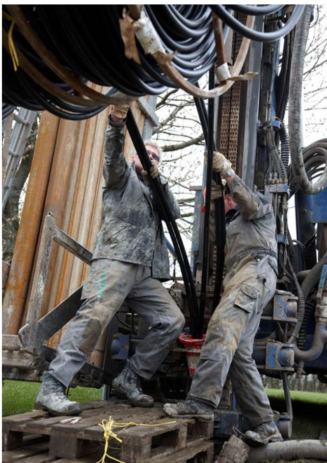
Figur 7.5. Installation af slanger/borehulssonder (double loop).
