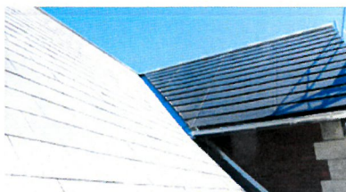
Building integrated PV into total renovation of old house in Hellerup with new windows and new roof.
