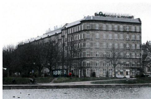
So-called Copenhagen roofs with PV on protected building Søpassagen has been a great success based on design by Solarplan.
