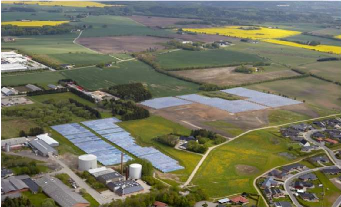
Fig. 6.13: Solar collectors and borehole storage implemented
