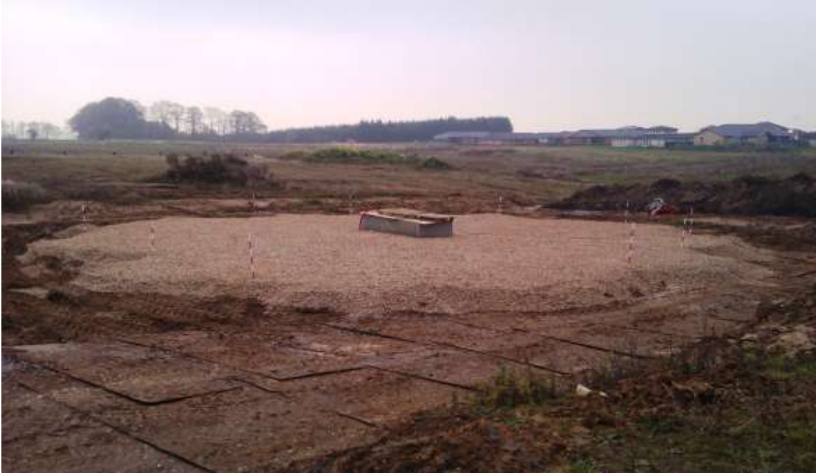
Fig. 6.7: Cockle shells in place
