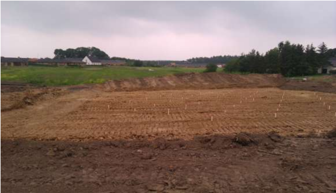
Fig. 6.2: The boreholes are placed
