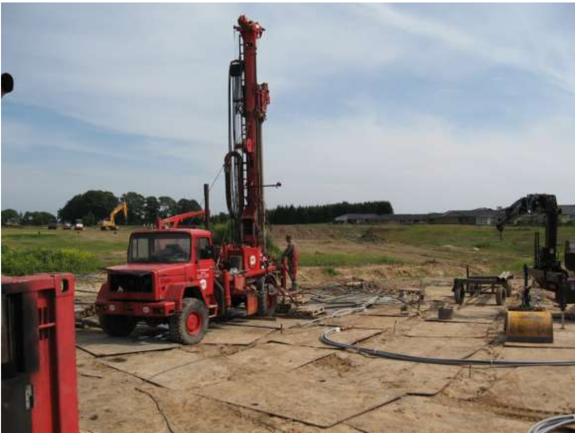
Fig. 6.3: Drilling of boreholes (1)
