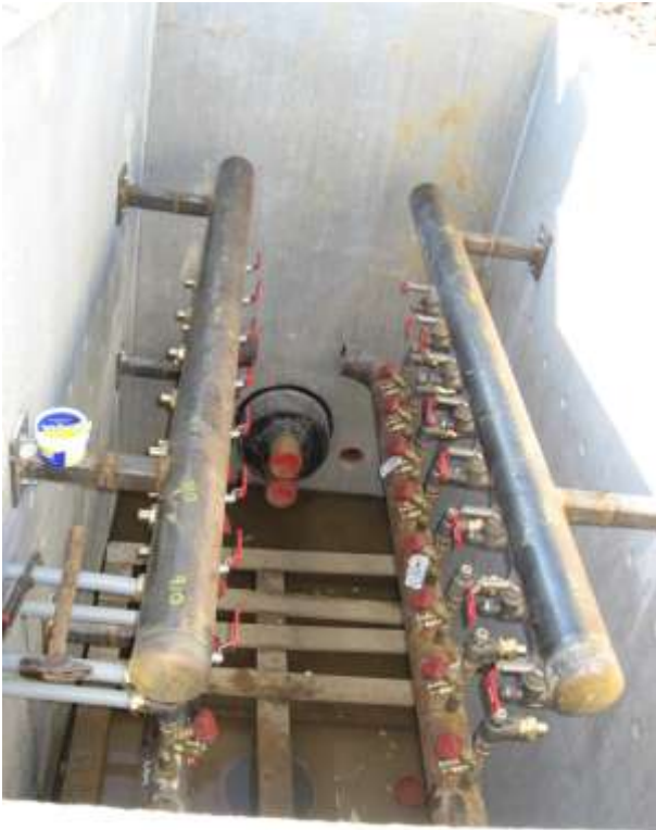
Fig. 6.9: Manifolds in well. Uninsulated left and connected and insulated right
