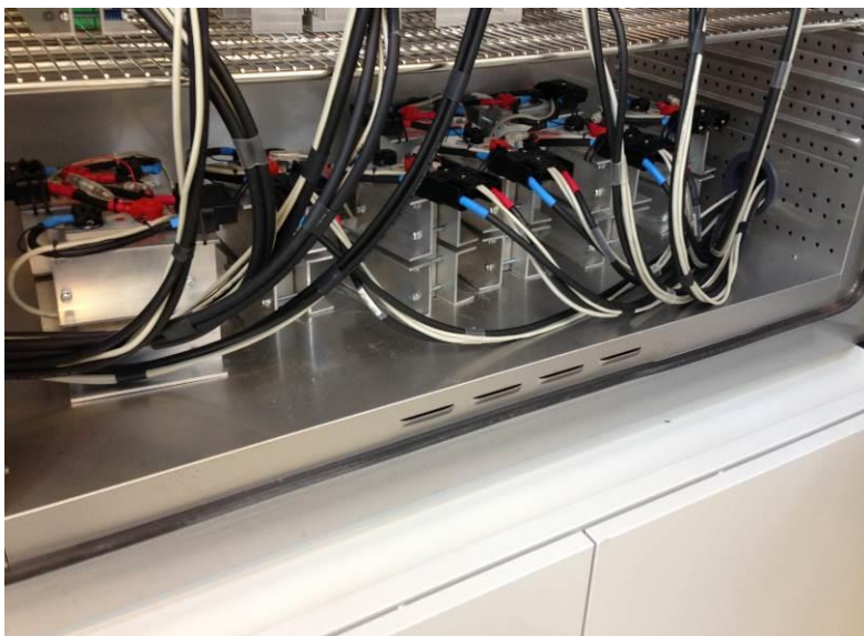
Figure 93: Pictures of some of the battery cells during test in test chamber
