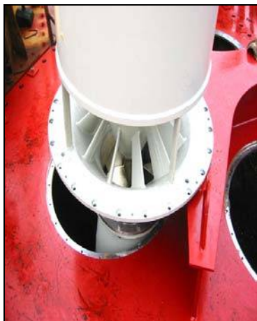
Fig. 3.15 Installation of draft tube
