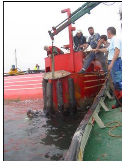
Fig. 5.4 Re-installation of fenders/fishtail plates at shoulder joint
