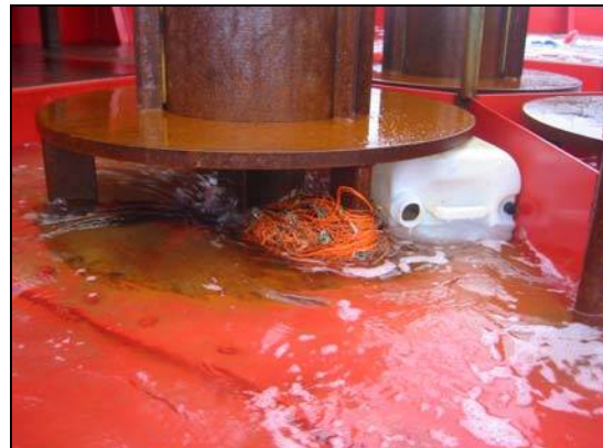
Fig. 3.4 Debris collecting at the dummy turbine cylinder gate
