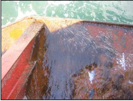
Fig. 8.1 Early moss growth on damper plate
