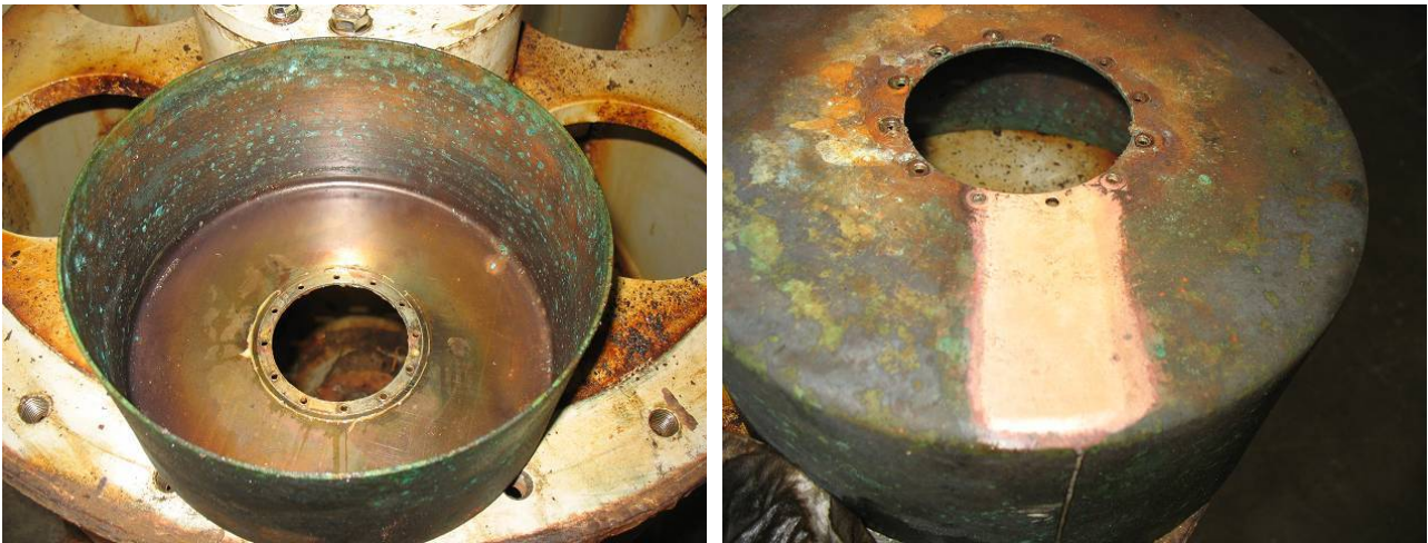
fig. 21: thrust bearing shield 2012
