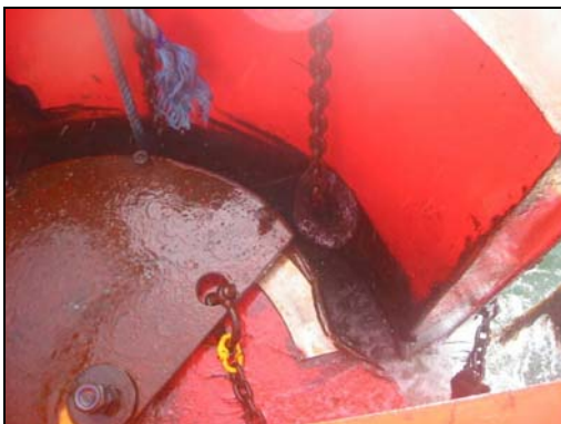
Fig. 5.13 Damage to port shoulder
