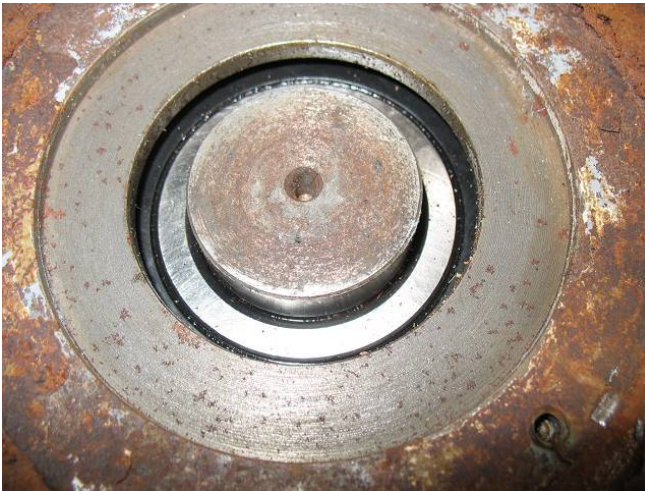
fig. 12: generator top and lower bearing
