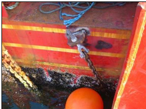
Fig. 5.23 Tensioning of fishtail plate
