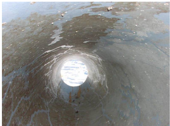
draft tube with Hempel anti-fouling paint
