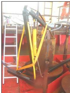
Fig. 3.8 Hoist used for dummy turbine removal
