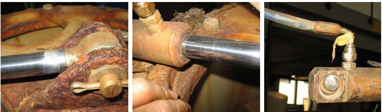
fig. 5: hydraulic cylinder for operating gate
