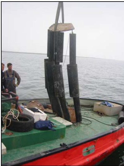
Fig. 5.3 Rubber fender/fishtail plate being loaded on to WD
