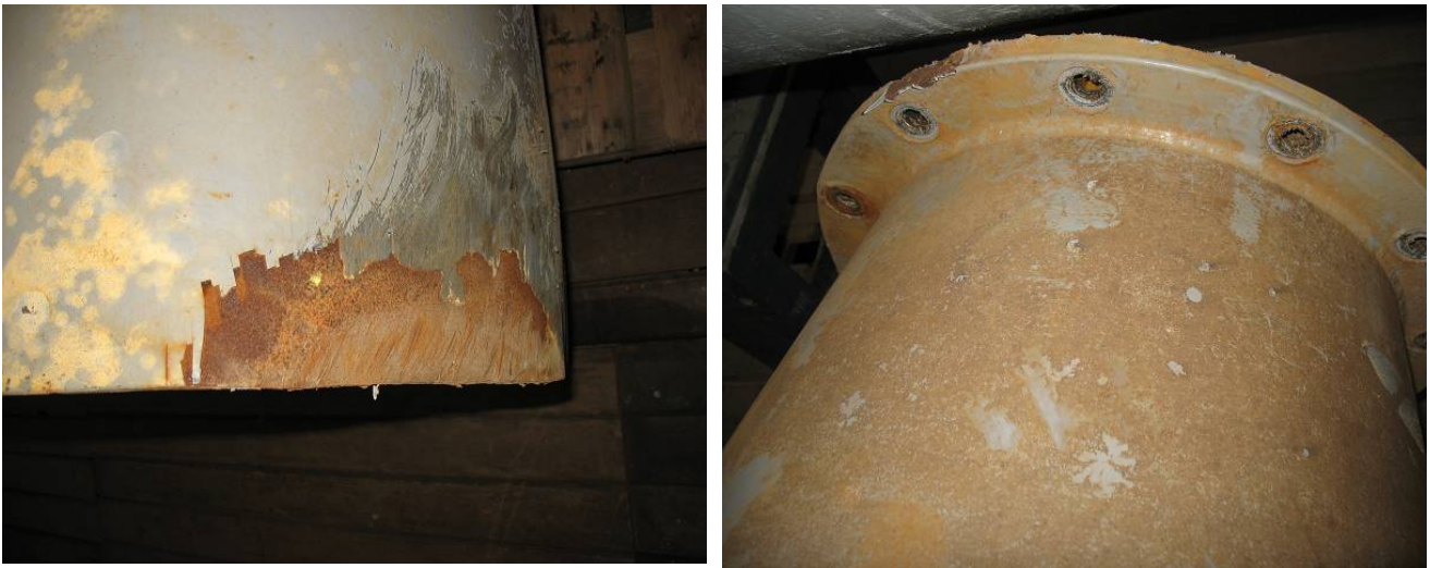
fig. 42: draft tubes with silicone paint system
