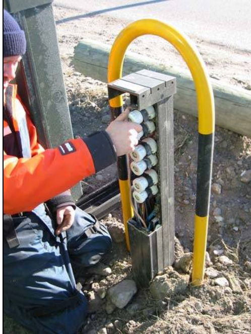
Fig. 1.1 Connection of WD to the grid
