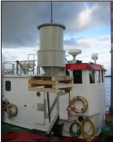
Fig. 3.11 Unloading of turbine centre section (runner & guide vanes)
