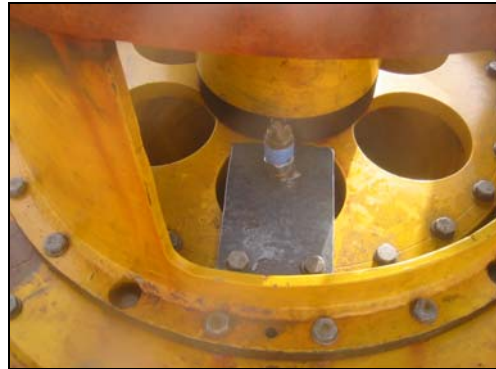
Fig. 3.2 Siphon turbine water level switch
