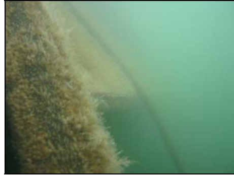
Fig. 8.2 Recent view of marine growth underneath the structure
