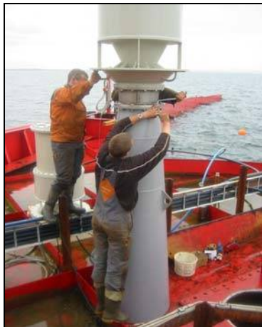
Fig. 3.13 Draft tube & centre section assembly
