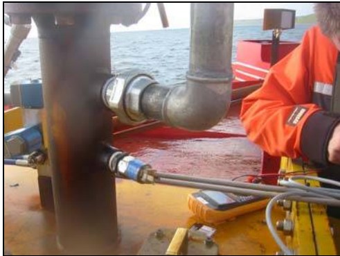
Fig. 3.1 Aeration tube water level switch installation
