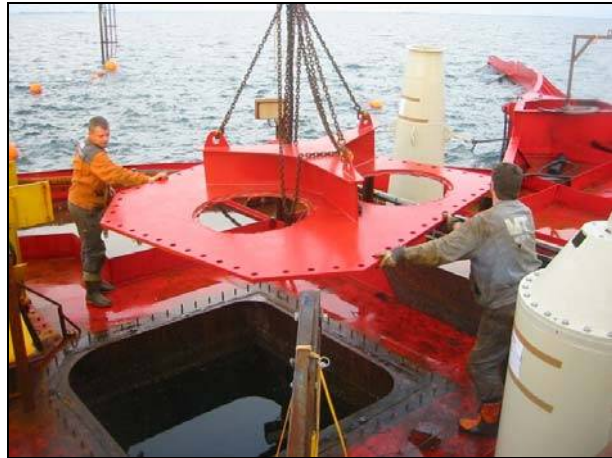
Fig. 3.12 Installation of floor plates
