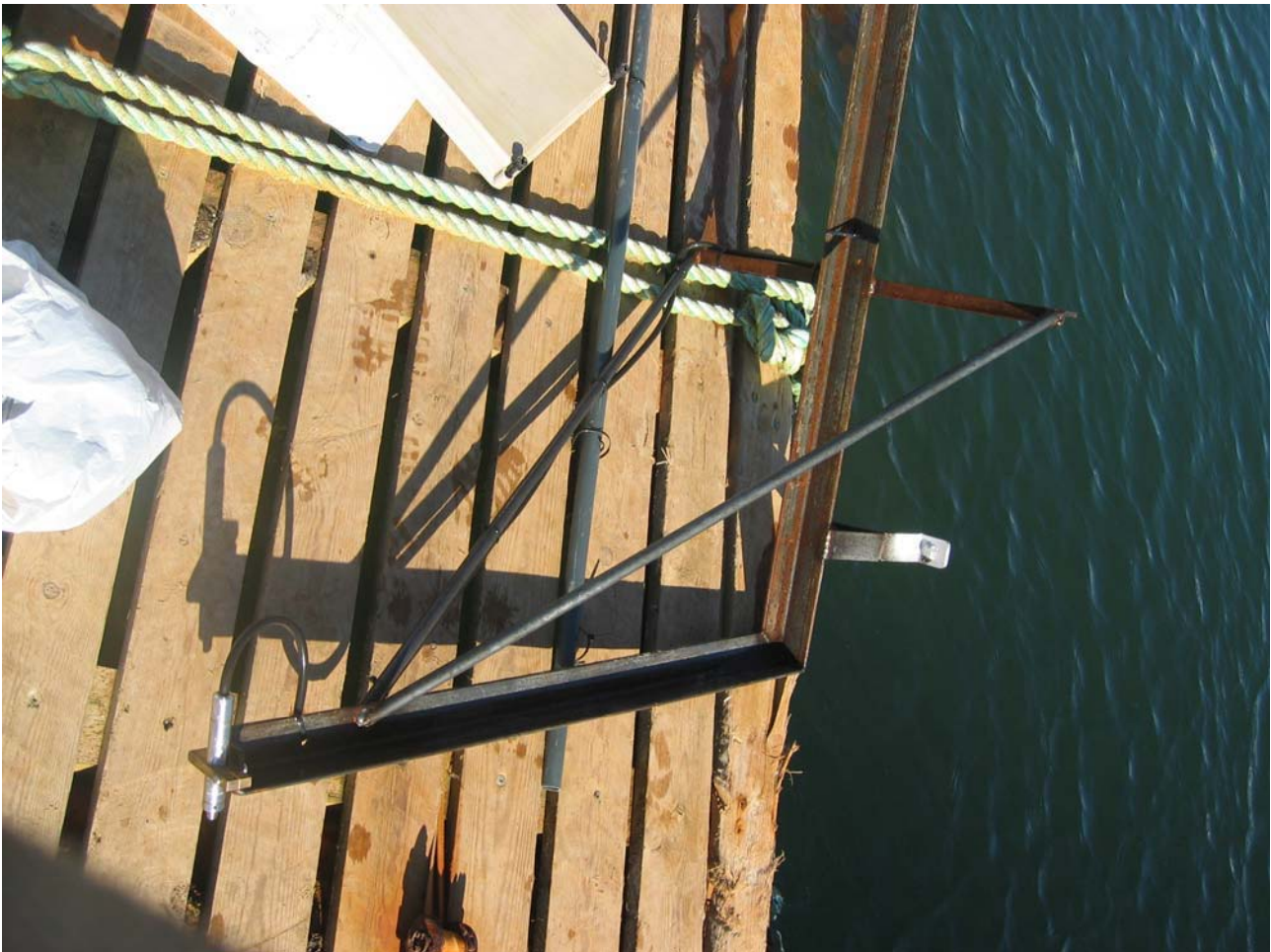
Figure 2.1: New pressure gauge on frame prior to installation on mooring pile.
