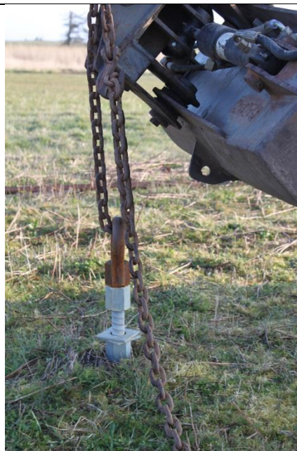
Initial pull test to 3 tons showed no movement. It only gives way sideways
