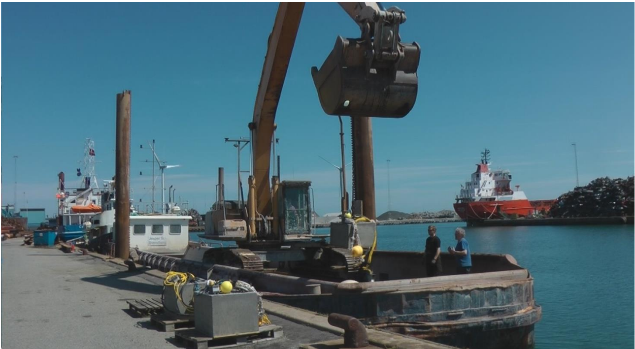
Anchor blocks lifted up onto boat
