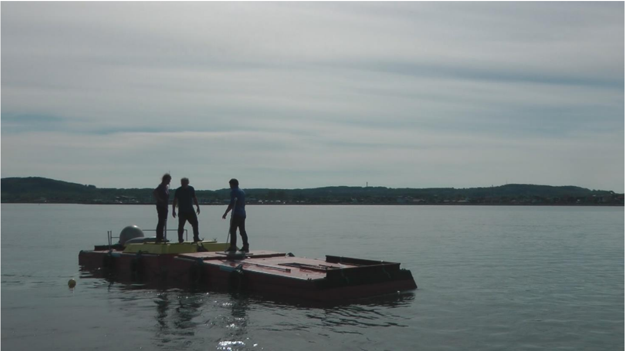
Quick on-site connections completed
