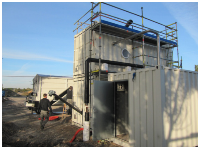
Picture 6: Installation in progress at Amagerforbrændingen.
