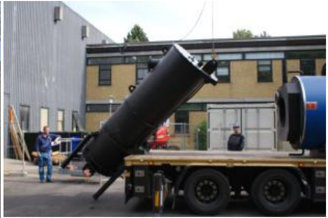
Picture 2: The gasifier is unloaded.
