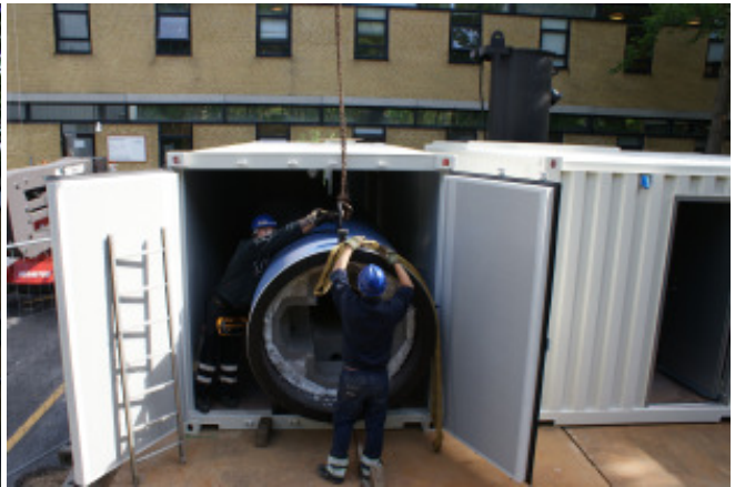
Picture 4: The combustion chamber is fitted in the container.
