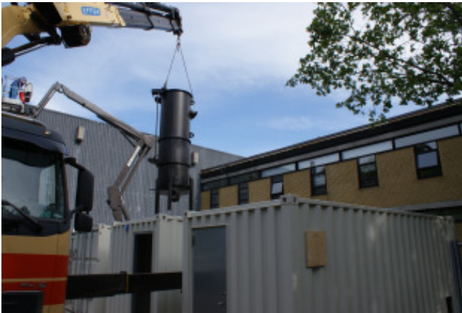
Picture 3: The gasifier is lifted into the container.
