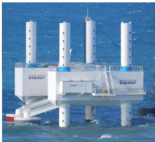
Fig. 3. Point absorber Wavestar prototype located near Hanstholm (DK) with two 5 m floaters and a floater arm length of 10 m. The main dimensions are: 32 m × 17 m × 6.5 m (L × W × H).
