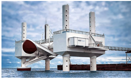
Fig. 9 Photo of Wavestar prototype with one floater on water surface ("production mode") and one lifted from water surface ("storm protection mode")
