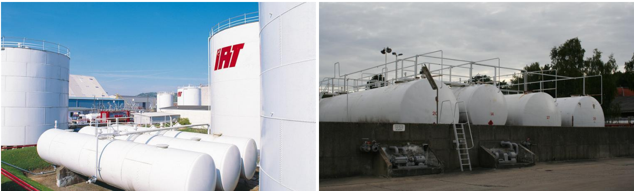
Figure 7: Tank capacity in Aabenraa
