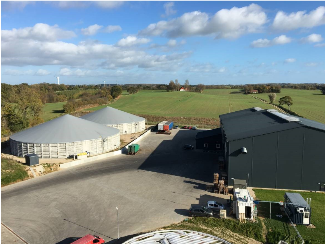
Figure 1: The picture is taken from top of one of the digestion reactors at Midtfyn Biogas (Nature Energy). The white 20' container in the lower right corner contains the electrolyser developed by GreenHydrogen. The blue container contains the gas-cleaning plant and the methanisation reactor developed by DTU MEK, Unicat Catalysts and Elplatek. The pipes and wiring between the containers and the biogas plant are also visible.
