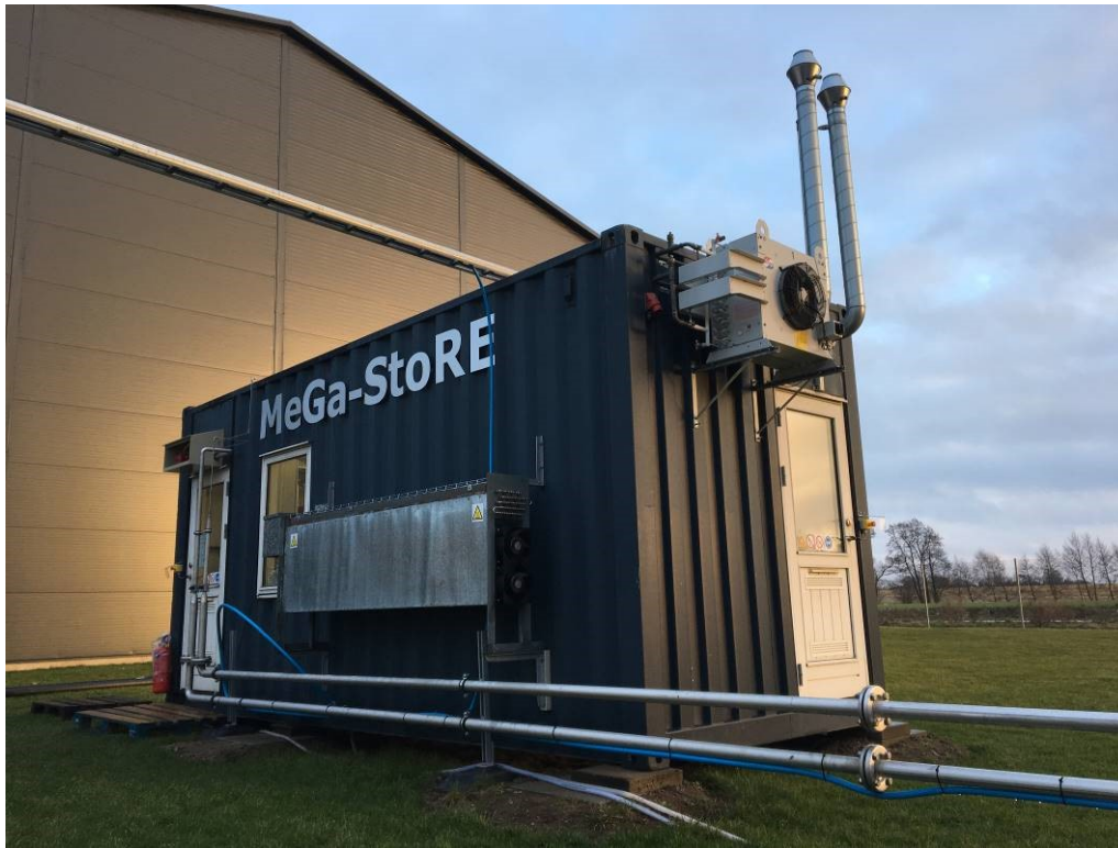
Figure 10: The container with the biogas cleaning plant and the methanisation unit from the outside. Hanging on the side, it is possible to see the heat exchanger for the oil cooling system. On the end there is a cooler for the compressor. In a future commercial system, the excess heat will be reused or recovered for e.g. district heating. Especially the excess heat from the methanisation reactor is of a high quality (above 200°C). It is also possible to see two 50 mm OD pipes. One pipe is the "dirty biogas" going into the container from one of the digesters at Midtfyn Biogas (Nature Energy). The other pipe is the clean and upgraded biogas going back to another digester. This is almost pure methane. Above the door (left) there is a small box containing the automatic shutdown valves that will close for the gas in case of alarm.
