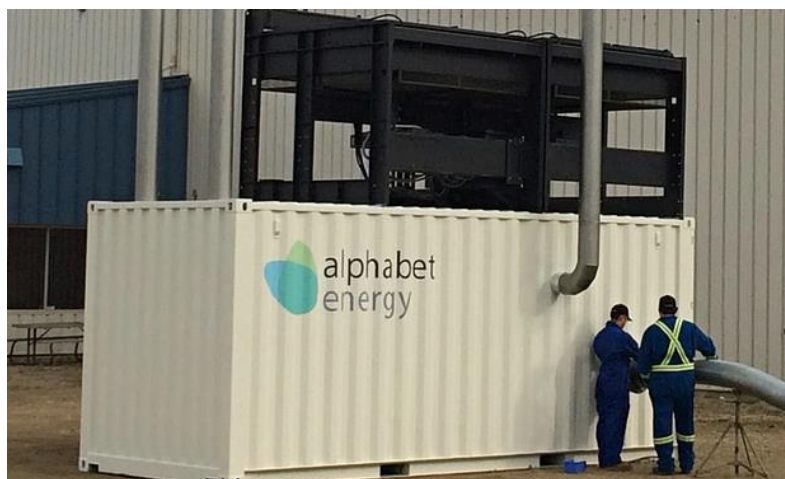
Figure 9 The Alphabet Energy's E1 25kW thermoelectric generator is housed in a standard shipping container, 16 or 20 feet long.
