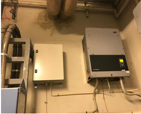
Photo 1. Setup of the RTU and measurement system at campus
