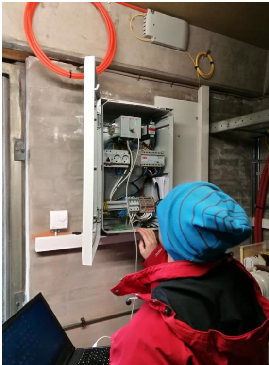
Photo 2. Setup of the RTU and measurement system in the 10/0.4-kV transformer station supplying the campus
