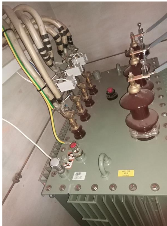
Photo 2. Setup of the RTU and measurement system in the 10/0.4-kV transformer station supplying the campus
