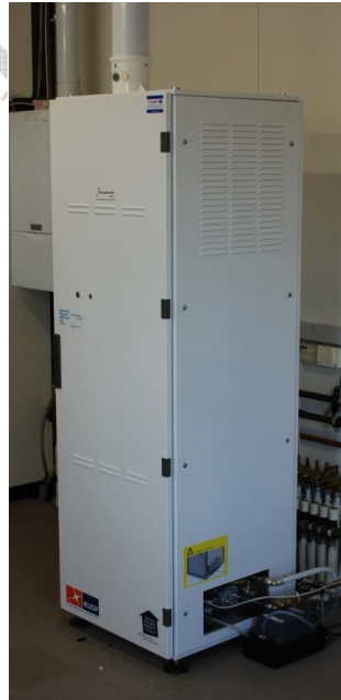
Figure 4: Dantherm Powers LTPEM system and selected performance data:
