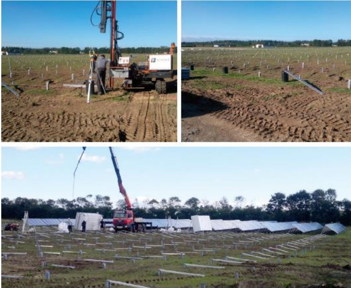
Fig. 13: Pictures from implementation of the solar collectors.
