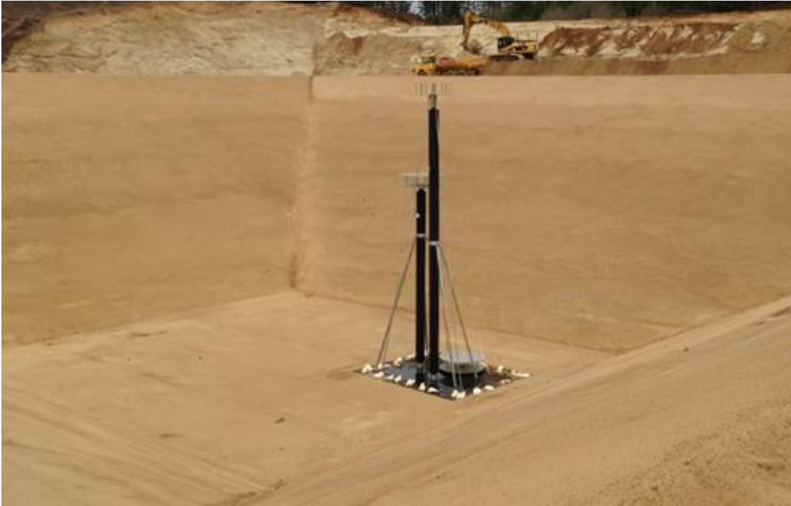
Fig. 10: In- and outlet with stabilization wires.
