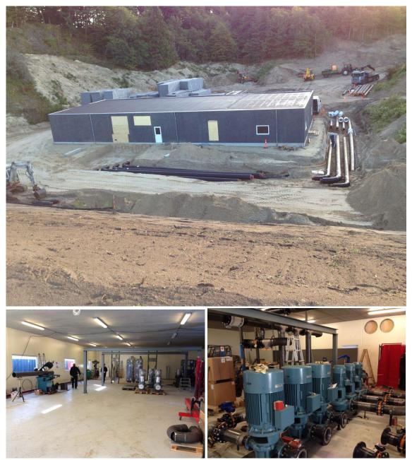
Fig. 15: Pictures from implementation in Lunderbjerg (Building, heat exchangers and pumps).
