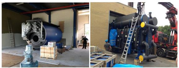
**Fig. 14:** Pictures from implementation in Søndervang (Boiler for absorption heat pump and absorption heat pump).
