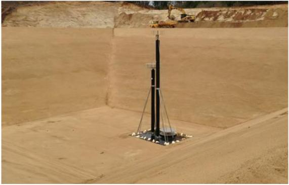
Fig. 10: In- and outlet with stabilization wires.
