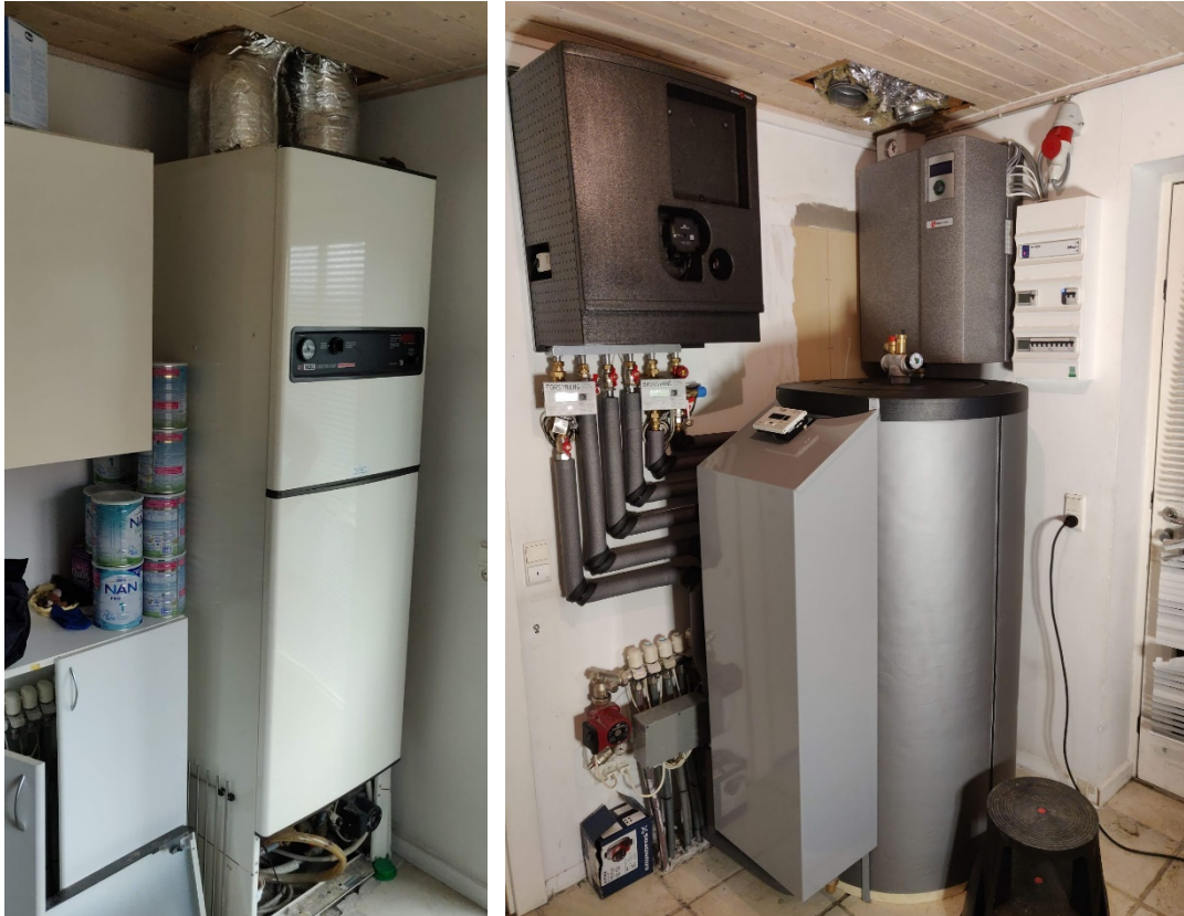
Figure 4: Before and after installation.
