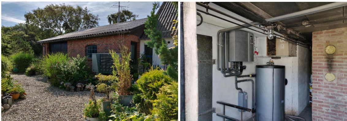
Suntherm/Alpha Innotec heat pump installed with local customer in Salling, Jutland, outside unit and inside storage and steering
