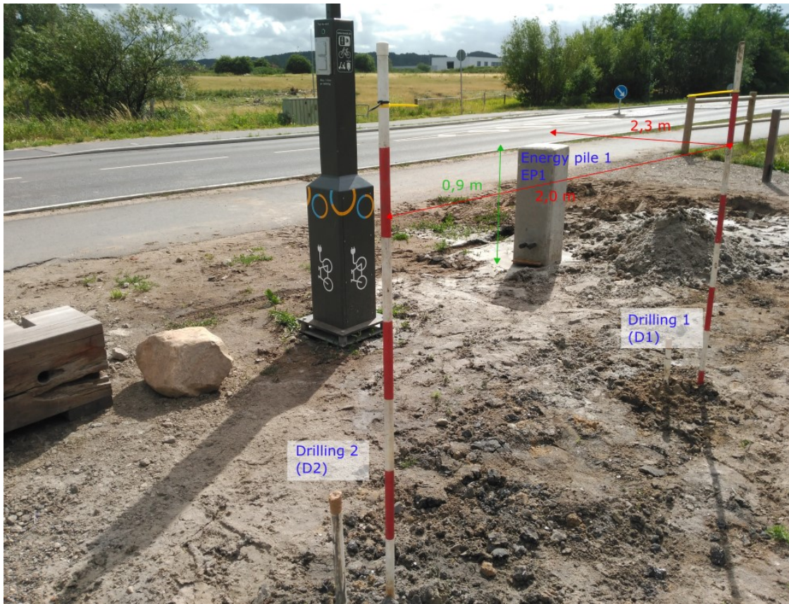
Figure 14: Energy pile 1 and the two additional drillings for the temperature sensors.
