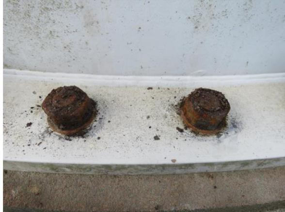
All foundations were inspected visual. More than 90% of the foundation is below ground, which means limited access! In one foundation, we found corrosion on foundation bolts. All other bolts were visual NDT inspected. No critical bolt-connections or welding's were found.
