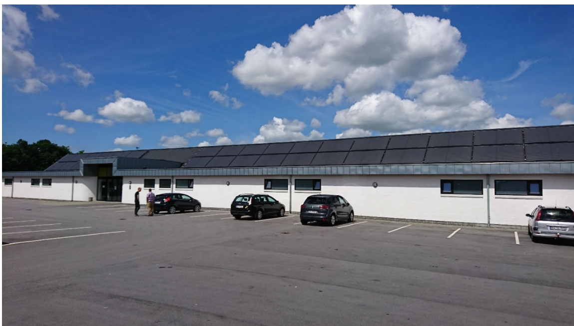
Figure 35. PVT system at Egeris Sports Center in Skive.
