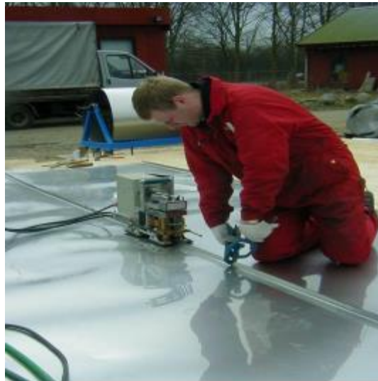
Figure 5. Induction welding of a stainless-steel liner [5]
