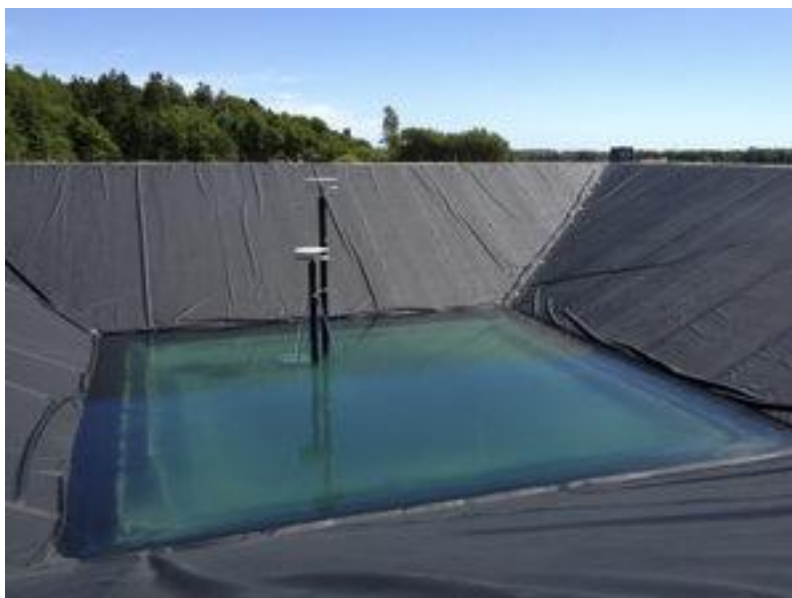
Figure 1. Picture of Dronninglund Pit Storage under construction. Dronninglund District heating; 37,573 m 2 of solar collectors and a 60,000 m 3 water in pit heat storage. (PlanEnergi)
