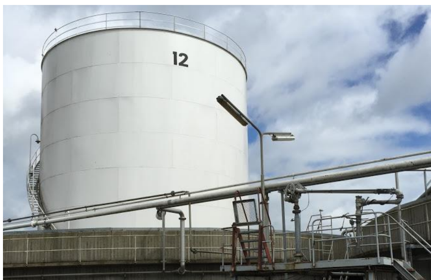
Figure 17 One of two Methanol tanks – each 2.500 m 3 - owned by Nordalim A/S, Port of Aarhus. The tanks are ISCC certified as warehouse for bio methanol traded by New Fuel A/S.
