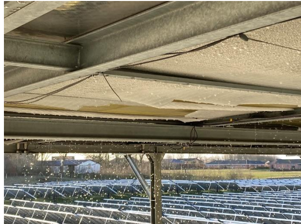
Icing of the evaporators
