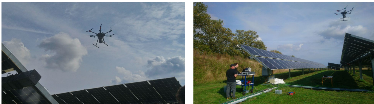
Figure 5.5.1 - Daylight drone during flight tests imaging Risø's PV farm. One operator is needed for the drone control and another one to control the image acquisition, the payload and the PV string modulation.
