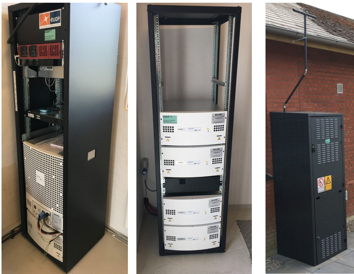
Figure 8 - Battery free system installation
