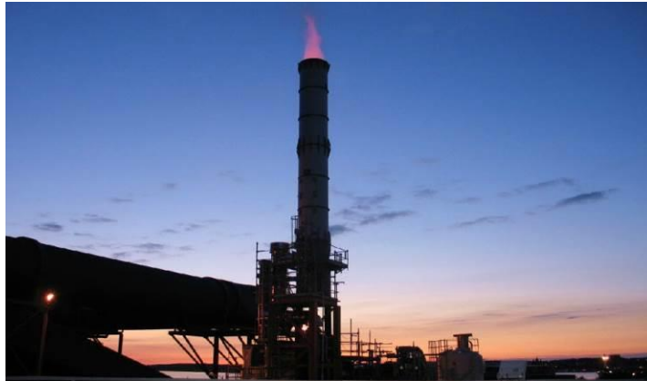
Figure 14: flaring of gas from the first operational campaign
