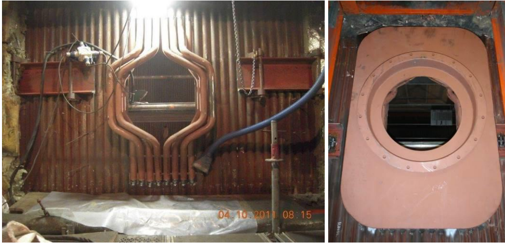
Figure 17: Modifications to the boiler
