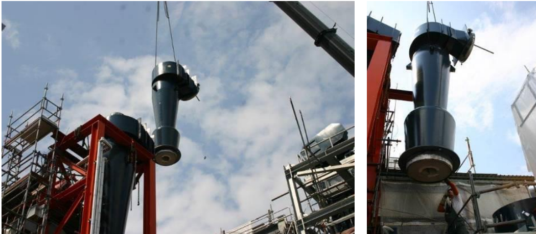
Figure 23: Installation of two new cyclones
