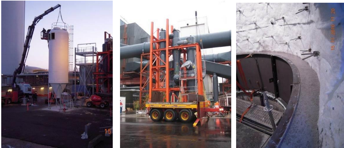
Figure 10: From left to right: silo installation; reactor installation; refractory installation
