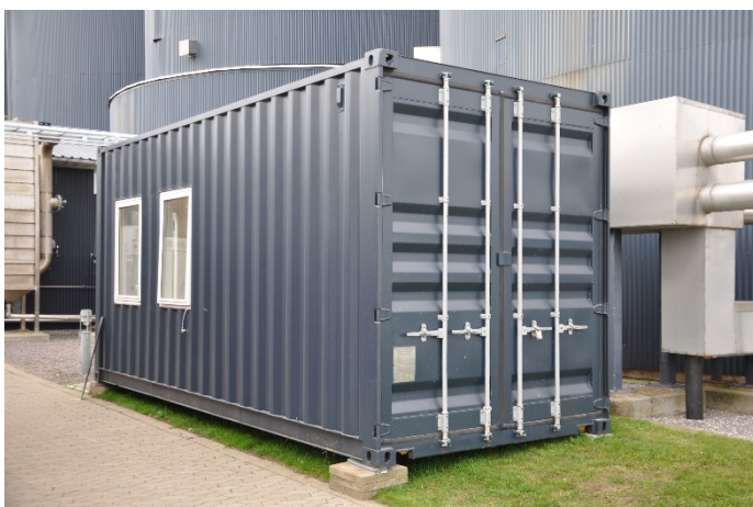
Picture 5 The container installed at Lemvig Biogas plant.
