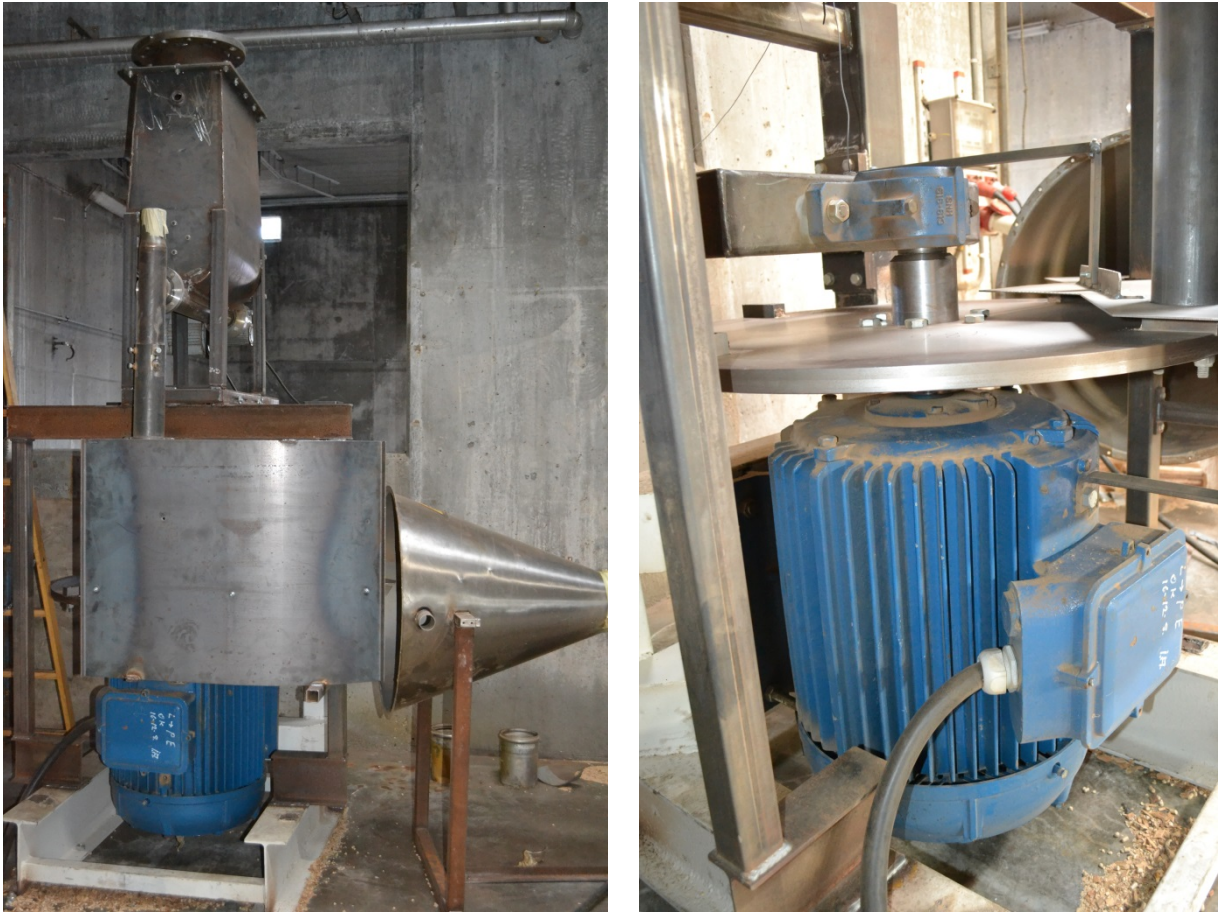
Figure 2. Pictures of the facility
