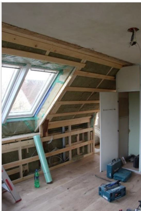
Figure 12 Renovation of the external wall and roof of the case study.
