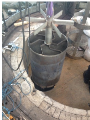
Picture 8 Installation of monolith
