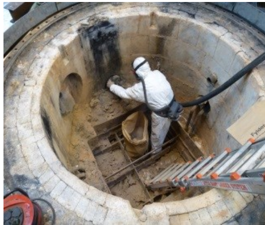
Picture 3 Change out of internals i.e. catalyst trays and internals I in very dusty environment
