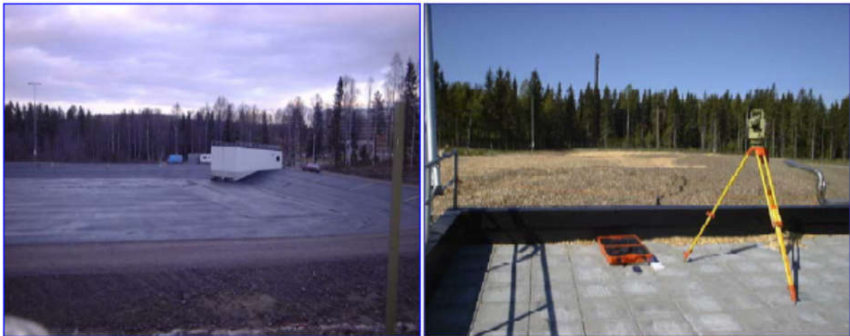
Fig. 3.3. The seasonal snow storage system in Sundsvall (Sweden). The pump house is the white constructed block (left), and the snow pile insulated with wood chips can be seen (right) [21].
