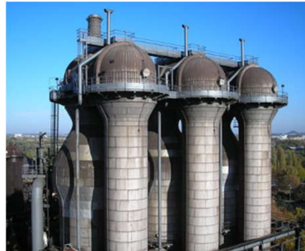
Fig. 4.4. Three Cowper stoves in operation at a steelmaking plant in Duisburg [42].
