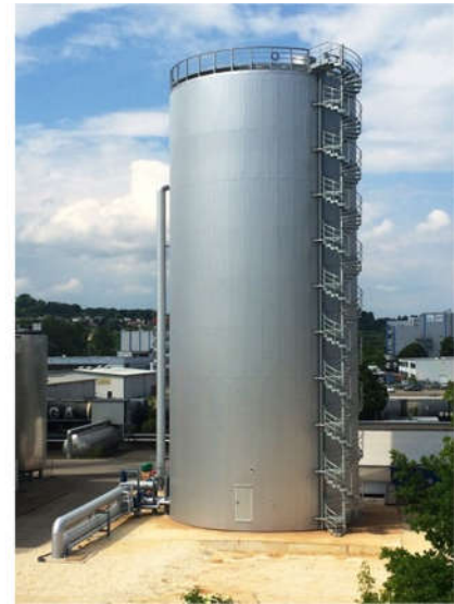
Fig. 2.6. Integration of sensible TES system into the district heating system located in Ulm, Germany [12].
