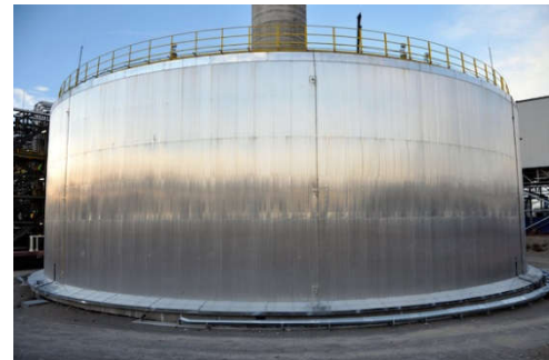
Fig. 5.2. Molten salt storage tank (© Solar Reserve).
