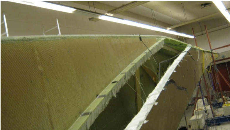
Figure 85 Damage of the adhesive bond near the root
