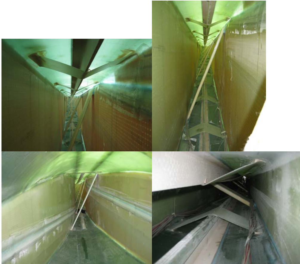
Figure 48: Photos from the inside of the assembled boxgirder.
