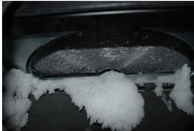
Figure 16: Even a rotary heat exchanger proved to be prone to icing issues when operated in a conventional manner.
