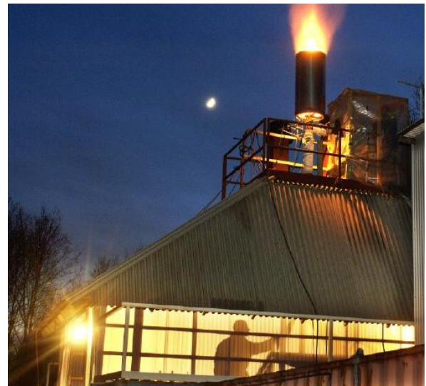
Figure 2: 500 kW LT-CFB test plant at DTU.
