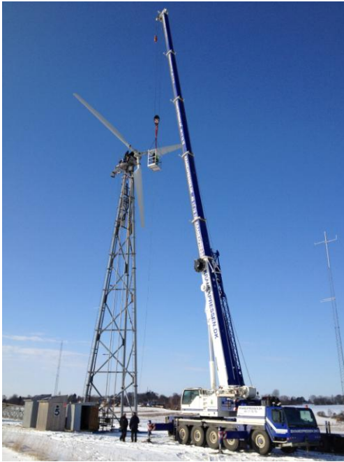
Figure 22 The rotor of the Tellus turbine at DTU Campus Risoe was taken down in March 2013 so that the turbine could be rebuilt to the rotating test rig shown in a sketch to the right.
