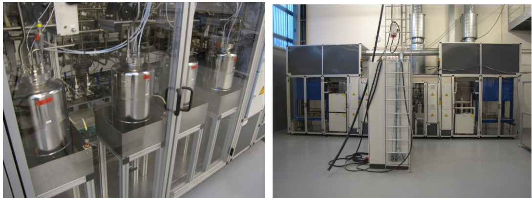
Figure: The fuel processing test facility after successful installation at TOFC.
