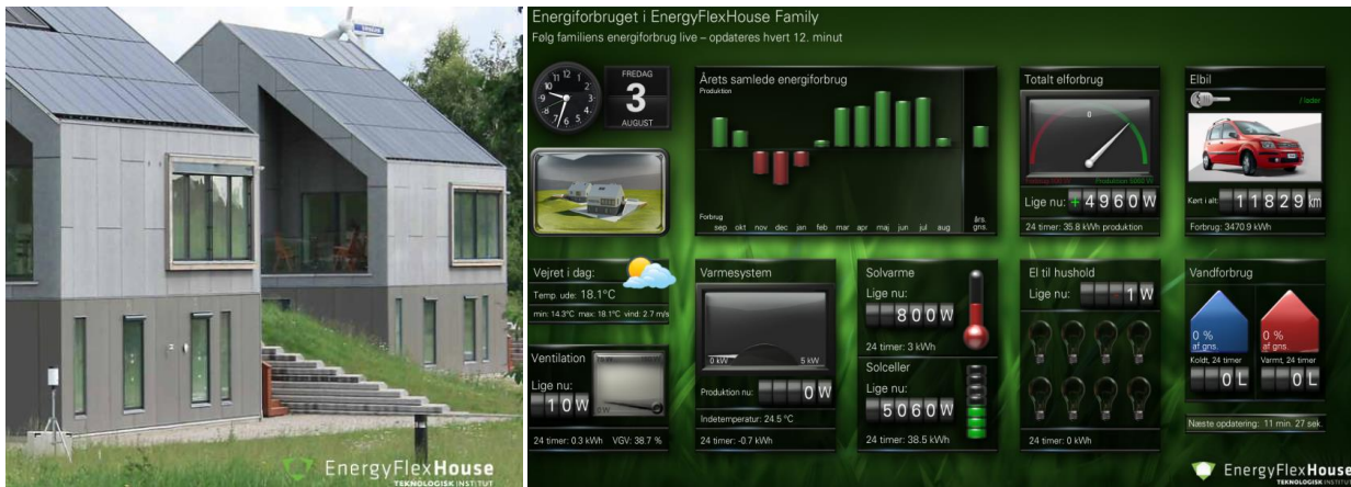
Figure 11: Energy Flex House consist of the lab-house (to the left) and the family house (to the right). The right panel is a screen shot of the on-line display showing real time actual energy flow in the Energy Flex Family House. https://www.youtube.com/watch?v=bFHWTLHh5G4
