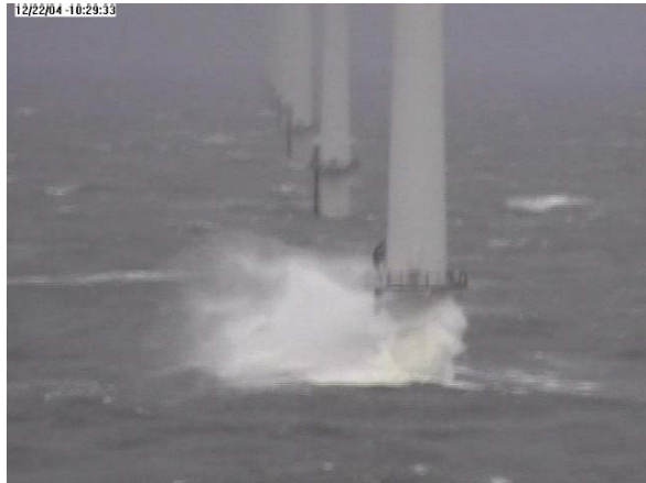
Figure 1: Example of severe run-up at a Horns Rev wind turbine, Vattenfall and DONG Energy.
