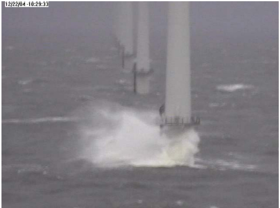
Fig 3.2 Example of severe run-up at a Horns Rev wind turbine. Photo by courtesy of Vattenfall and DONG Energy
