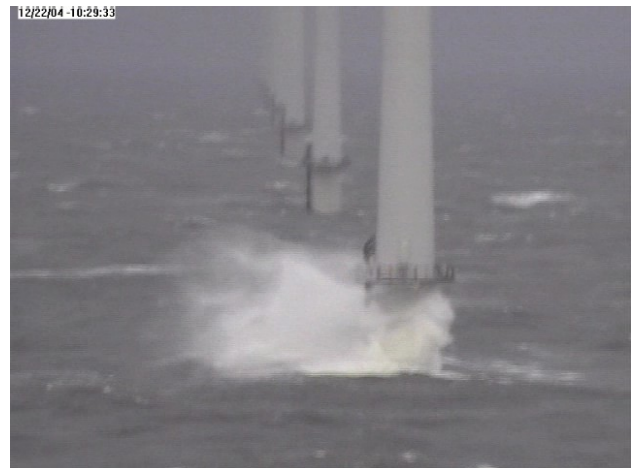
Figure 1 Example of severe run-up at a Horns Rev wind turbine, Vattenfall and DONG Energy.
